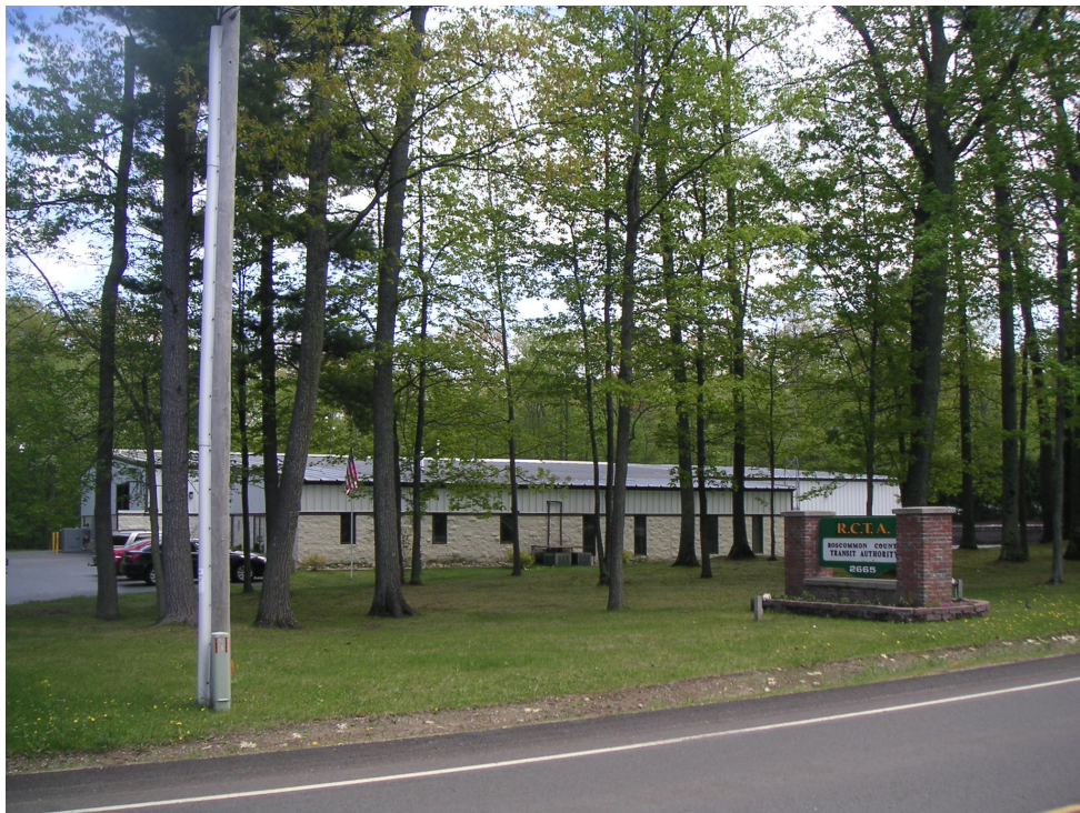
RCTA facility near Prudenville (Source: KFH Group)
